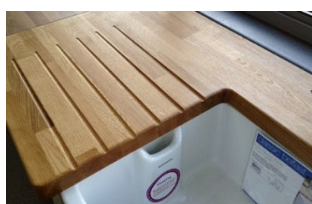
Belfast sink cut-out with drainer grooves
